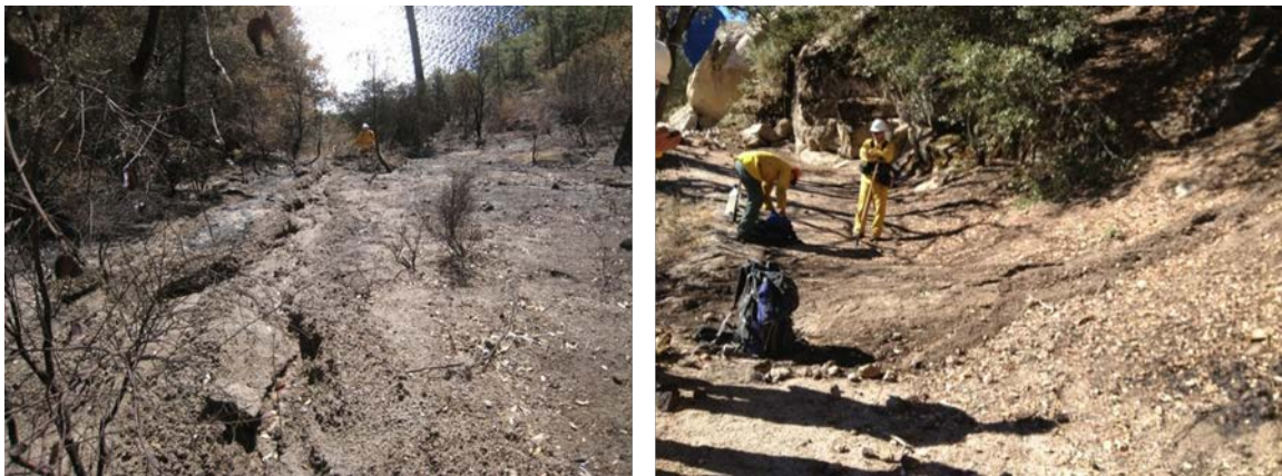
Figure 5: Rill formation (left) on the North side of Hetch Hetchy and subsequent sediment deposit (right) on the Beehive/Vernon Lake trail.
