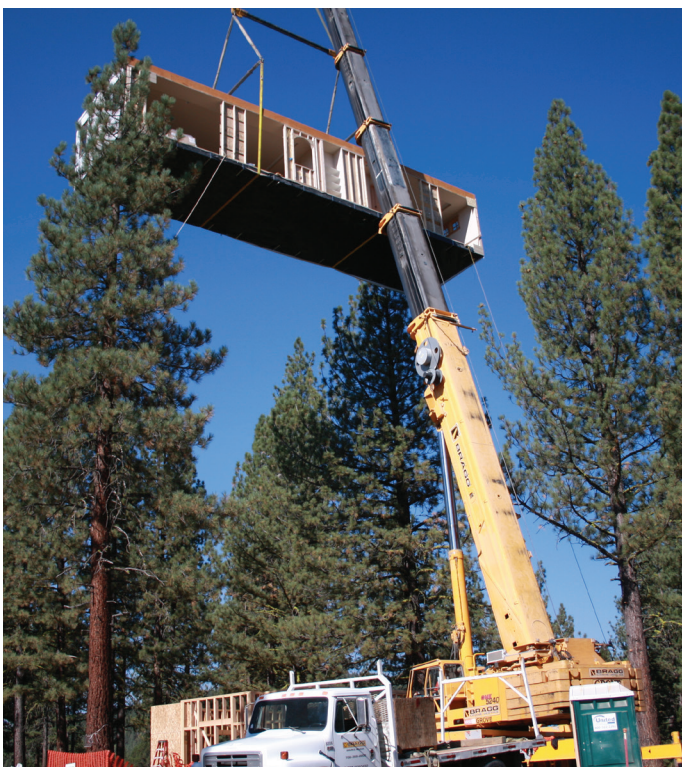
A Factory-Built Housing dwelling unit being installed by crane.
