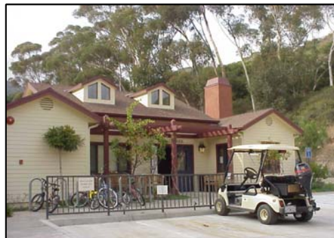
Constructed in 2002 Bird Park apartments includes 24 units for very low income families
