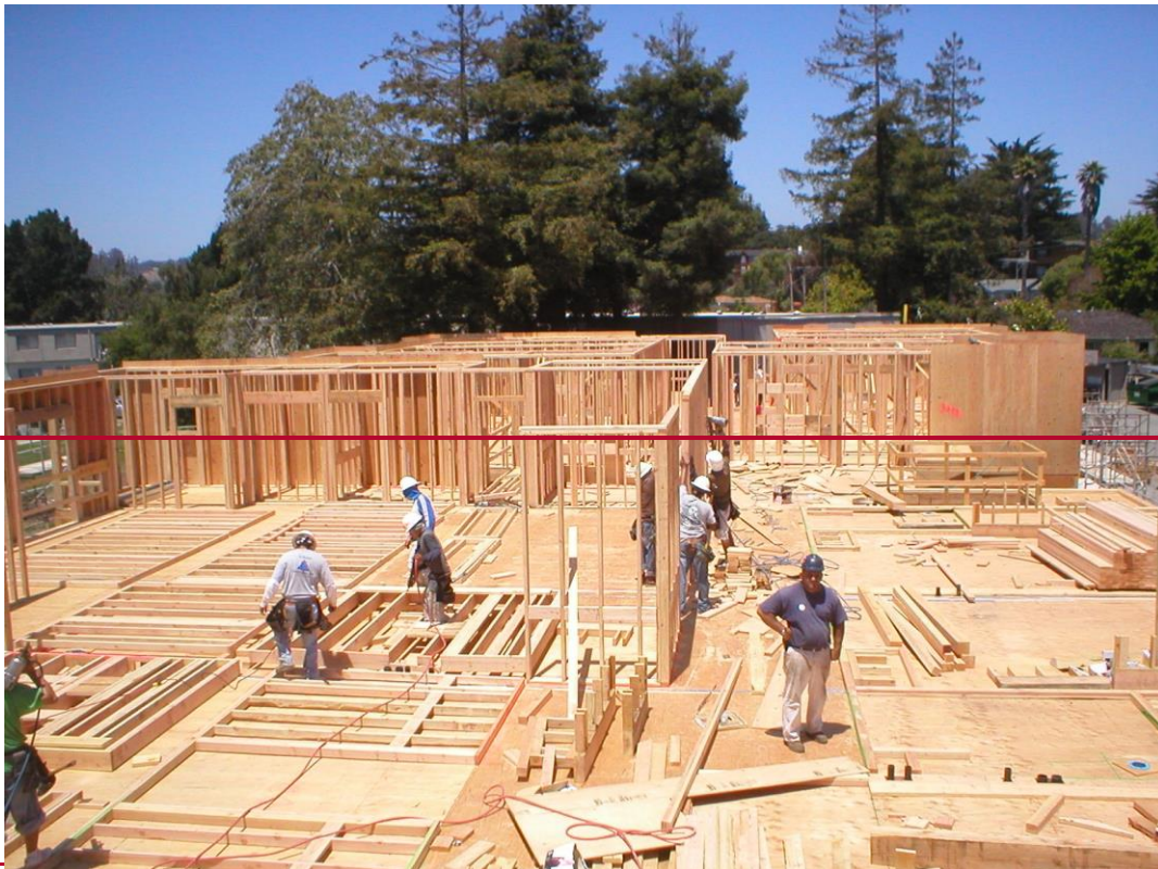
Construction at 750 Bay Avenue
