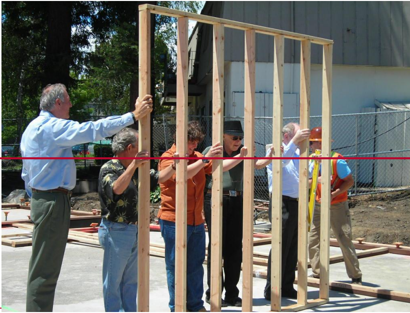
City and First Community Housing officials celebrate at Bay Avenue Senior Apartments wall raising ceremony June 5, 2009)
