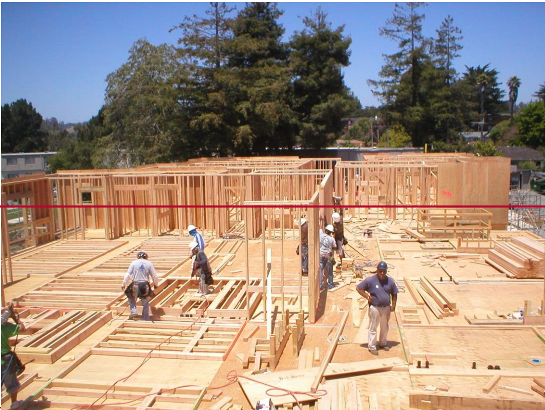
Construction at 750 Bay Avenue
