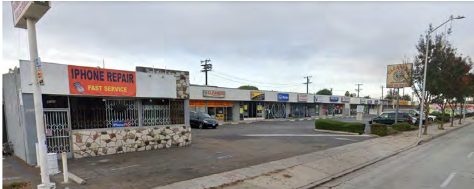
Imperial Highway near Lakewood Boulevard
