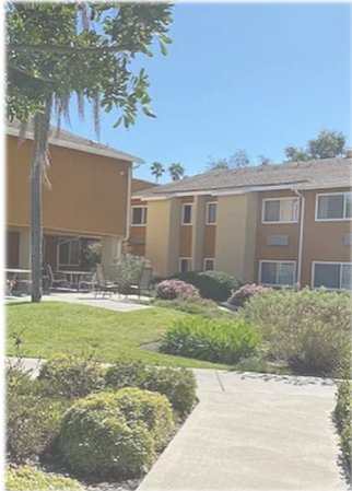
Good Shepherd Homes Rehabilitated Housing
