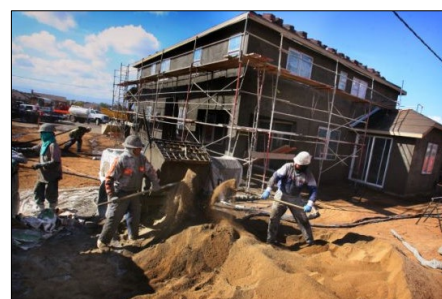
Figure 5-4: Housing construction in Jurupa Valley
