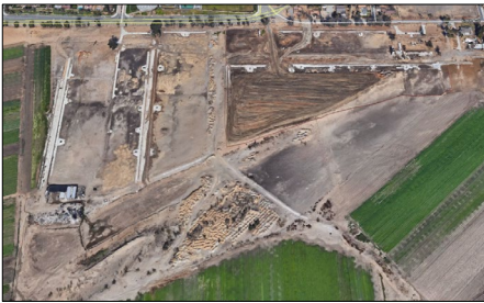
Figure 5-2: Subdivision under construction, Jurupa Valley
