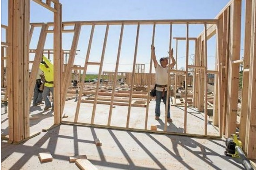
Figure 5-1: New housing construction in Jurupa Valley
