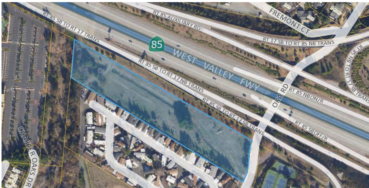
Figure D-26 Caltrans Right of Way (Site E-3)
