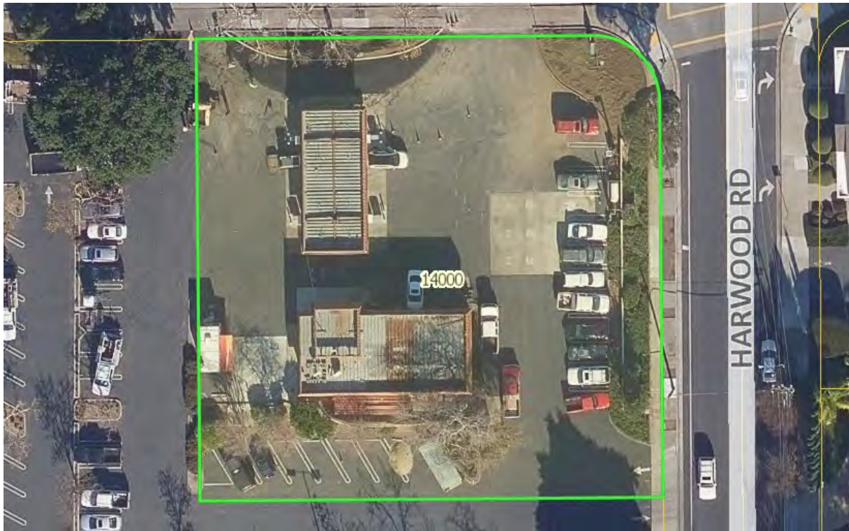
Figure D-33 Valero (Site H-1)
