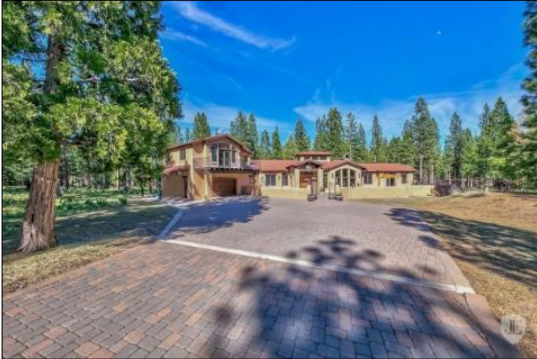
Photo AD-3. Home in Calpines in Modoc County
