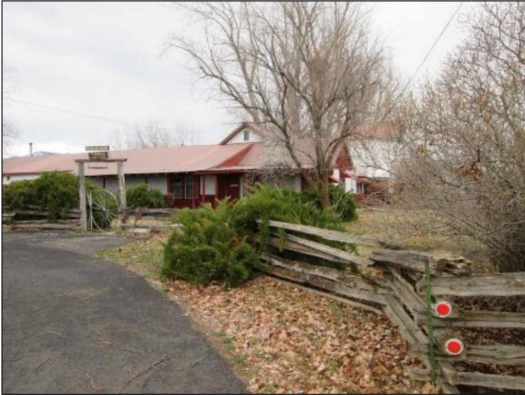
Photo AD-5. Rural Residential House in Modoc County
