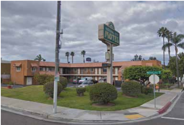
510 National City Blvd
