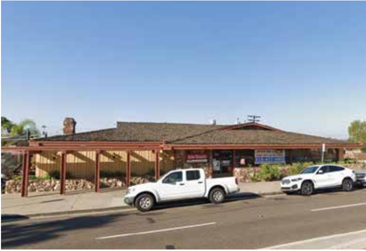
214 National City Blvd
