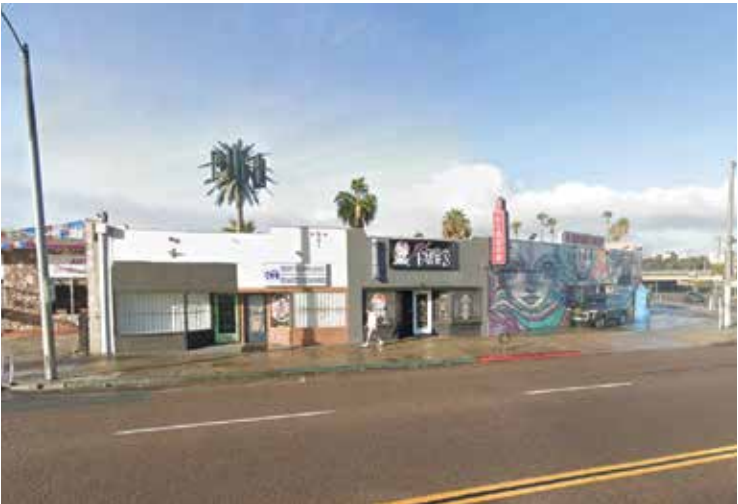
122 National City Blvd
