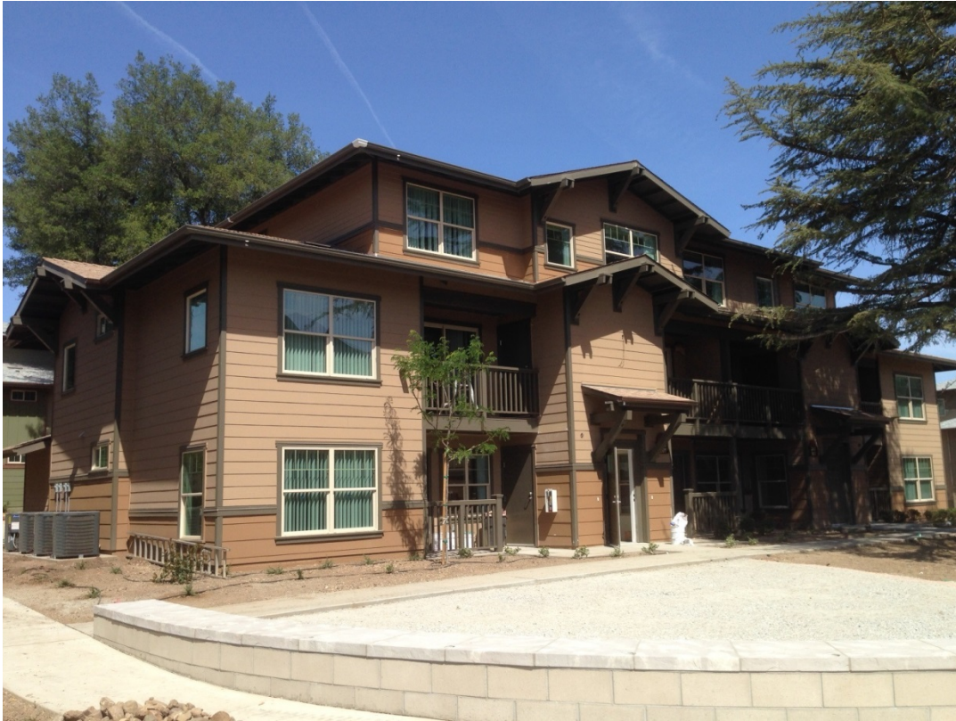
Oak Park Redevelopment, Phase One – Nearing Completion
