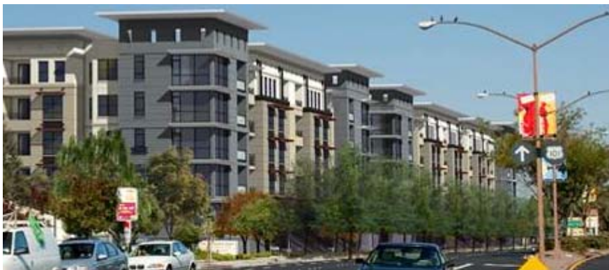
Radius Apartments, constructed in 2014 on Veterans Boulevard, include 22 low-income units in exchange for a density bonus.
