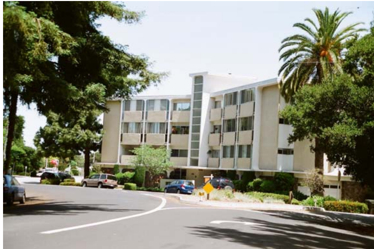
Multi-family residential building on Wellesley Crescent
