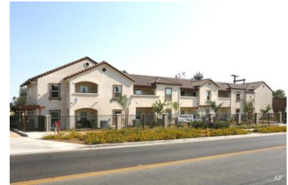
Grand Villas Senior Apartments
