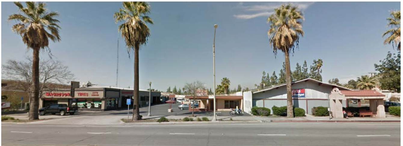
View of Site looking north from University Avenue
