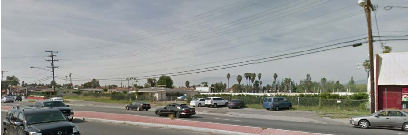
View of Site looking northeast from location near the intersection of Arlington Ave. & Van Buren Blvd.
