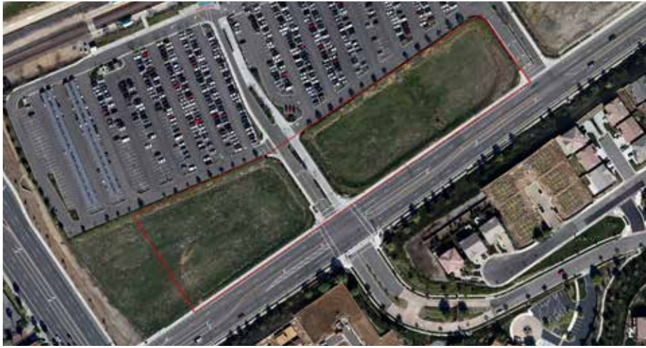
Site location and prior use
