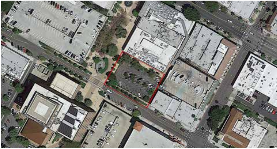
Site location and prior use
