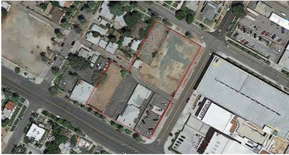
Site location and prior use
