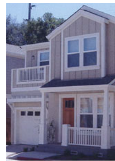
Manufactured Multifamily Home Courtesy of CMHI
