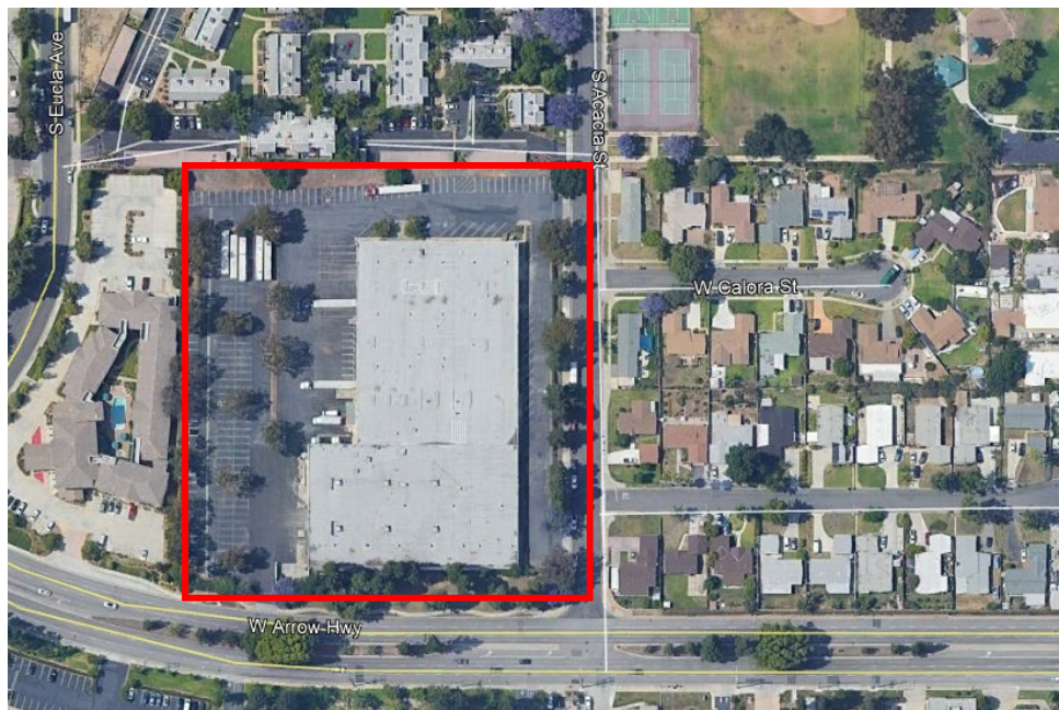
Figure A-8 Warehouse Site
