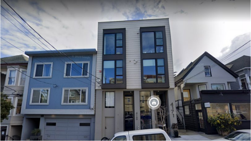
After Construction: February 2022
