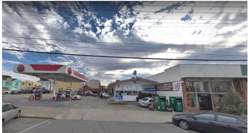
Before Construction: November 2017
