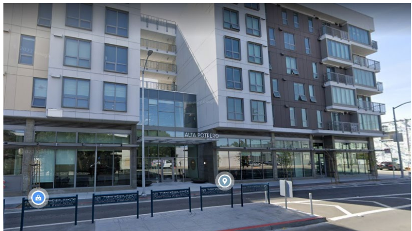
After Construction: April 2022
