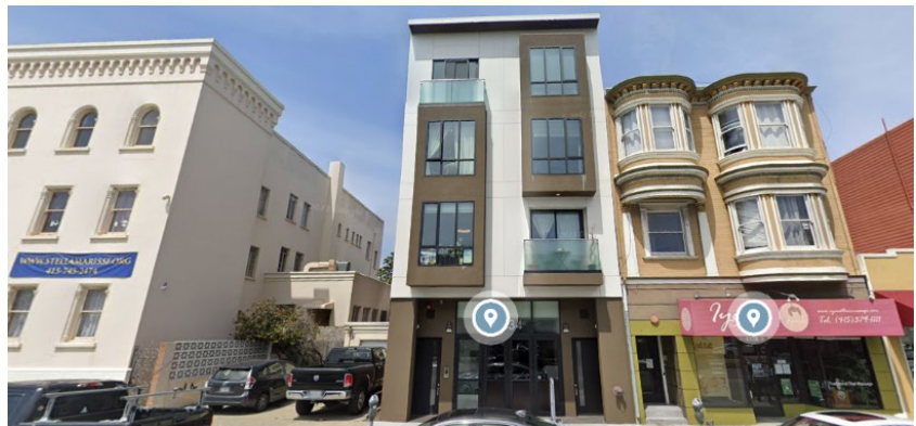
After Construction: April 2022
