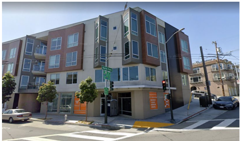
After Construction: April 2022
