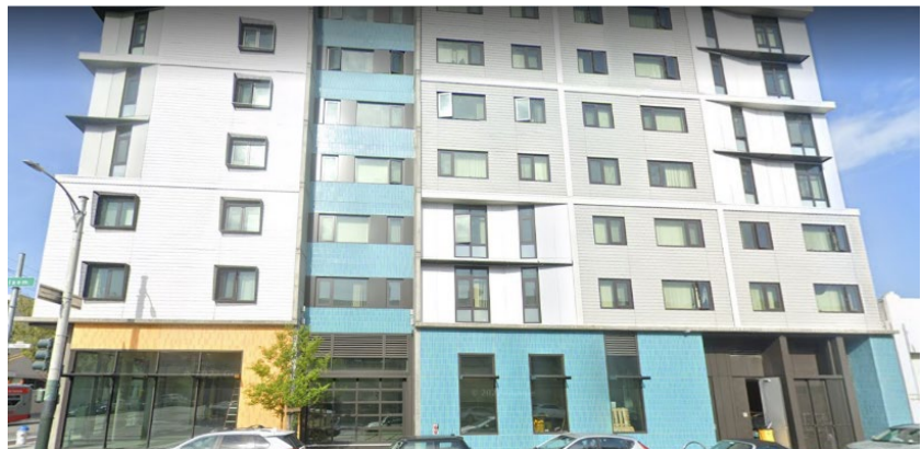
After Construction: April 2022
