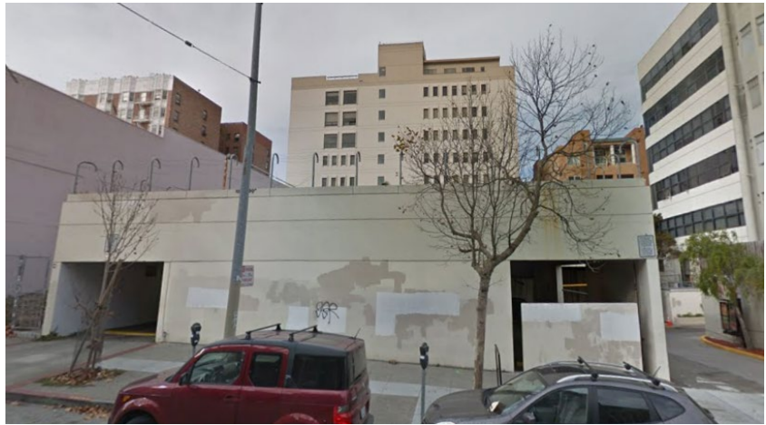
Before Construction: November 2013
