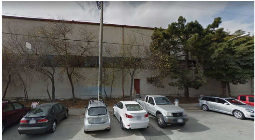
Before Construction: November 2013
