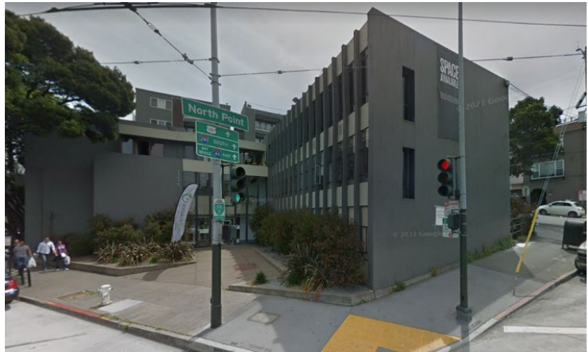
Before Construction: May 2014
