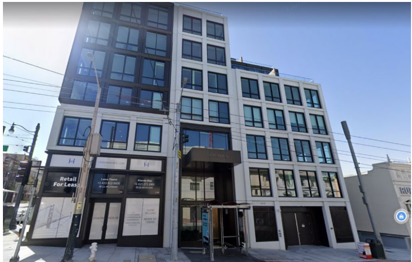
After Construction: April 2022
