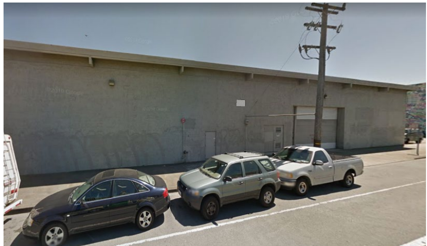
Before Construction: May 2013
