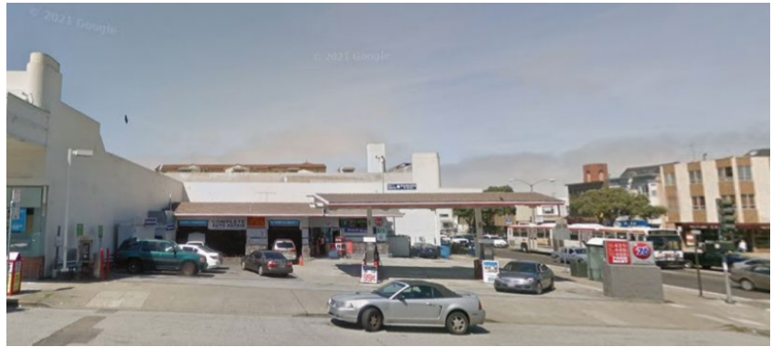
Before Construction: May 2011
