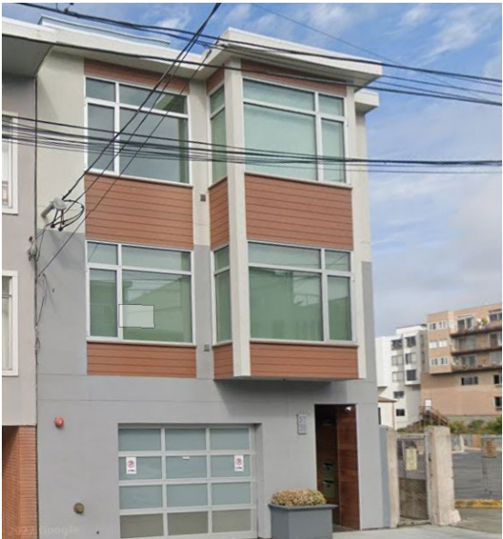
After Construction: January 2022
