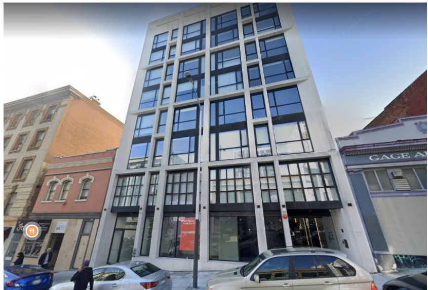
After Construction: April 2022
