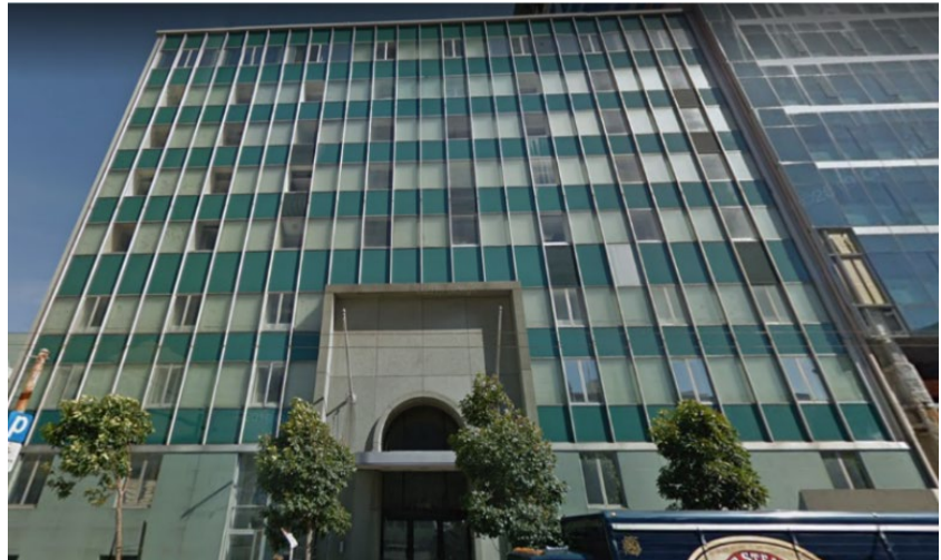
Before Construction: May 2014
