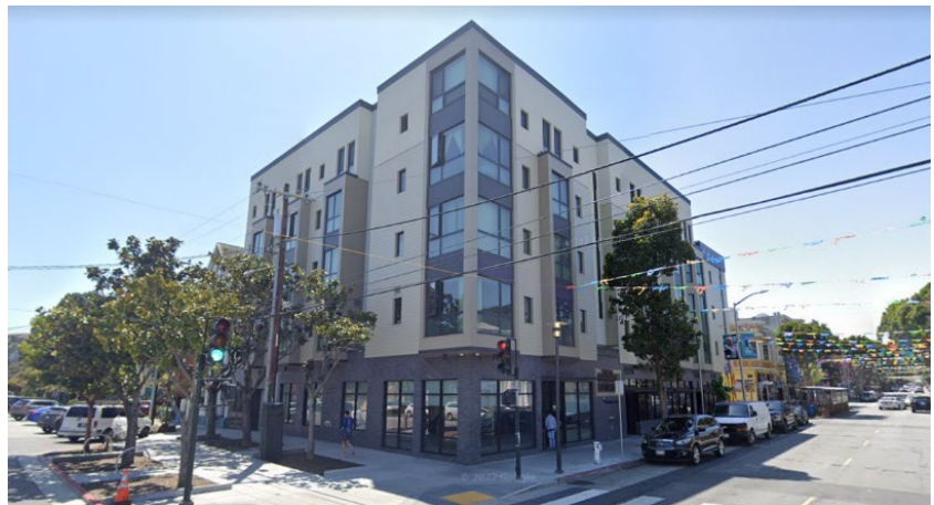
After Construction: April 2022
