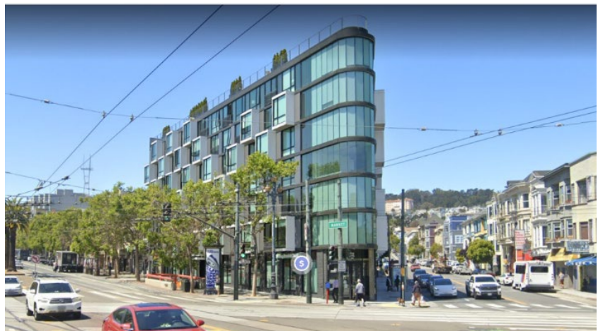
After Construction: May 2022
