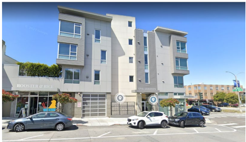
After Construction: April 2022
