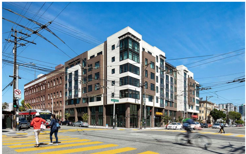
After Construction: July 2022
