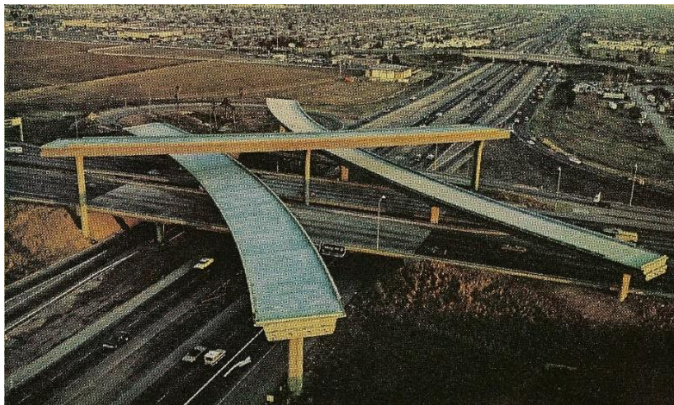
Figure 10: The 680, 280, and 101 freeway interchange, under construction in 1976
