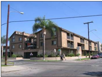
Recent Acquisition and Rehabilitation Project
