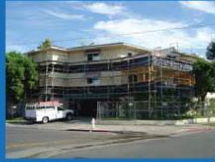
Sixth Street Rehabilitation
