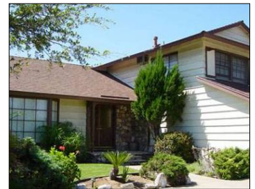
Community Care facility
