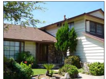
Community Care facility
