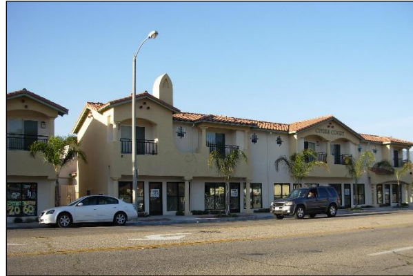
Citrus Court Apartments Mixed Use Project
