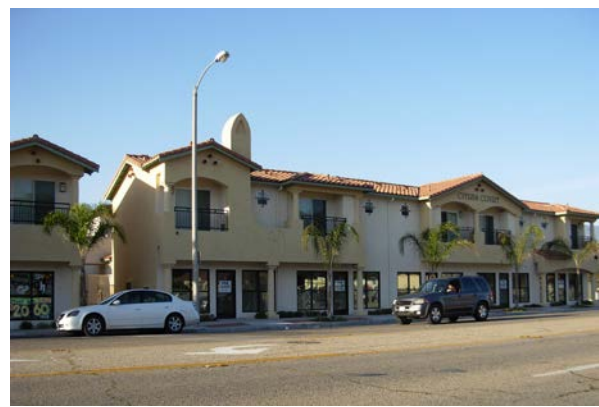
Citrus Court Apartments Mixed Use Project
