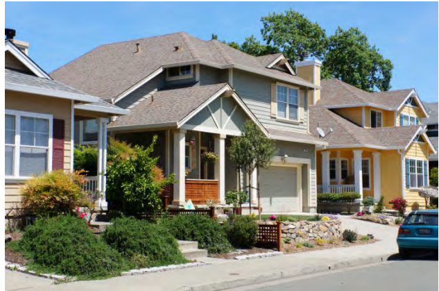
Single-family detached housing is one of the many types of housing available and envisioned in Santa Rosa.
