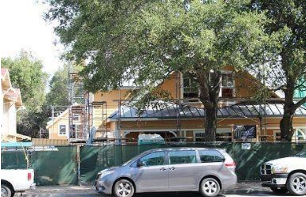
Mixed-use development under construction in Saratoga Village
