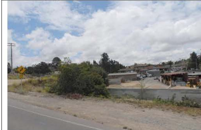
Materials yard consisting of small buildings, shade structures, and open yard storage (viewed from Monte Vista Drive looking south)
