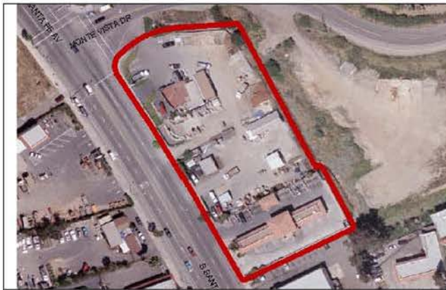
Above parcels are within Planning Area 1b (PA-1b) of the Downtown Specific Plan
