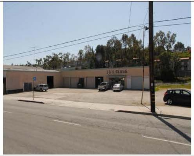
Looking west (from S. Santa Fe) at the glass installation contractor and open parking lot
