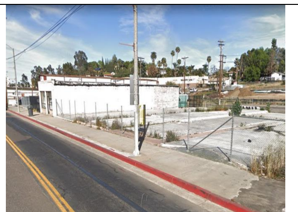
Existing commercial buildings along S. Santa Fe Avenue
