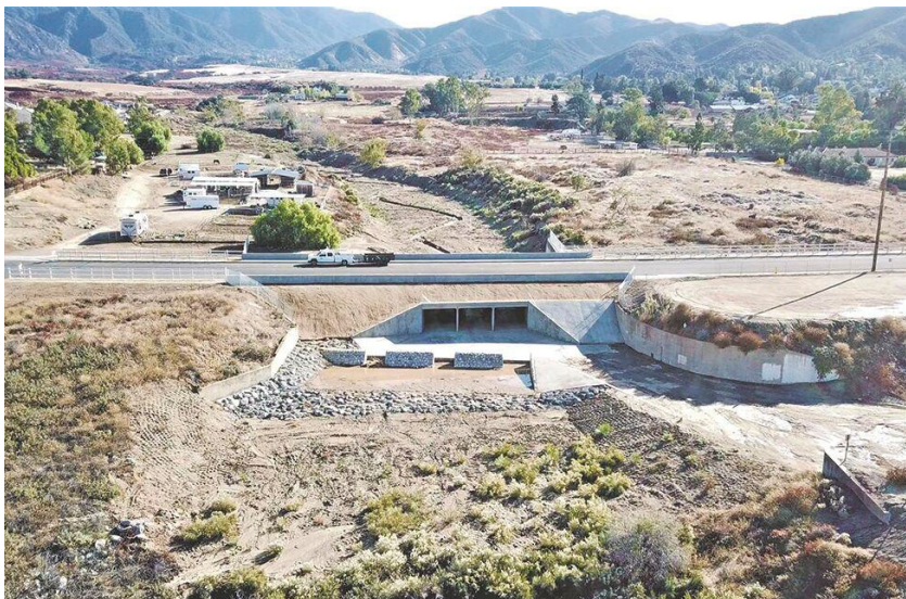
Grant funded low water crossing
