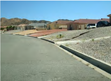
A neighborhood with curbs, gutters and paved roads.
