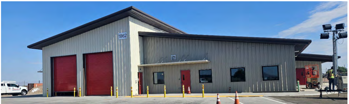
County of Imperial Seeley Fire Station and Cooling Center, Photo Credits: County of Imperial
