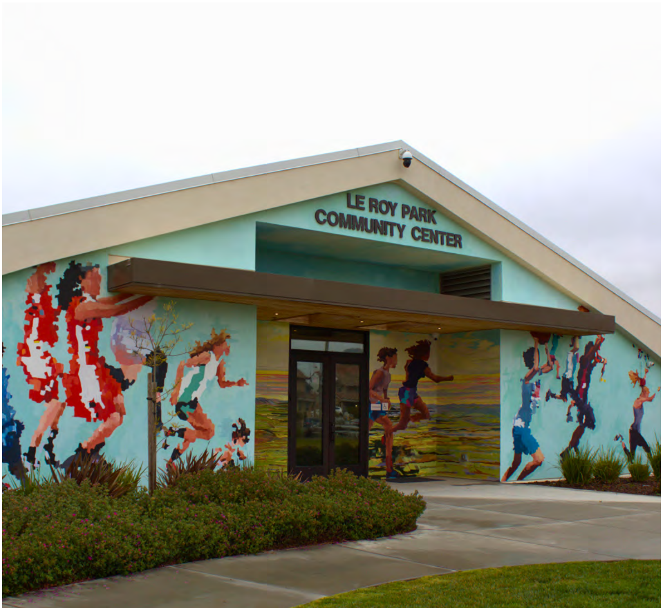
City of Guadalupe Le Roy Park Community Center, Photo Credit:Dayanira Cruz
