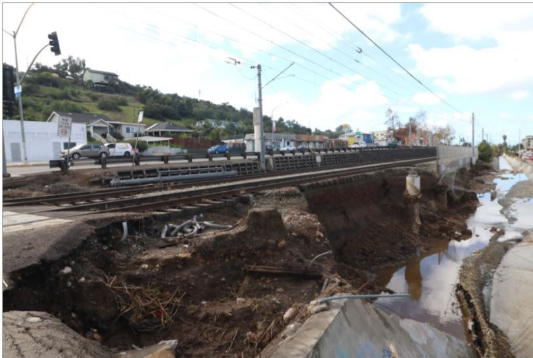
Figure 7: Damage to the Orange Line light rail in the Encanto neighborhood
